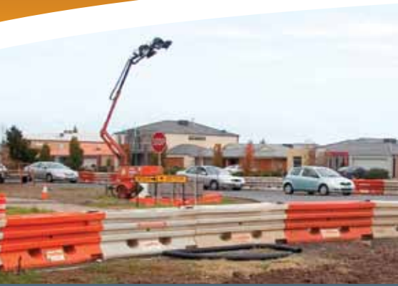
Motorists are encouraged to take care when travelling through roadworks.
