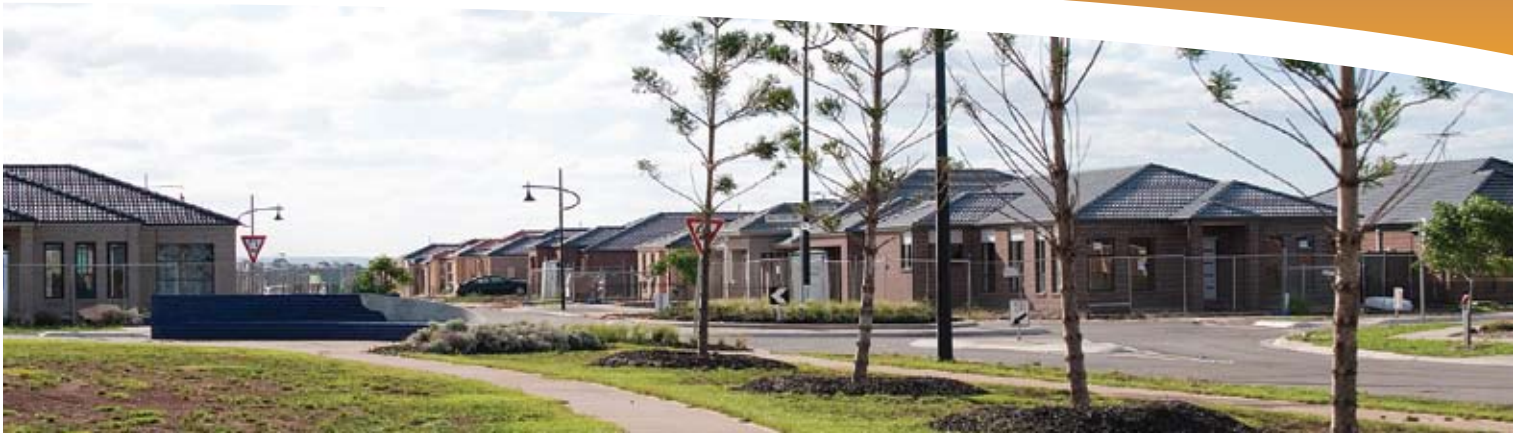
New homes under construction off Eagleridge Promenade.
